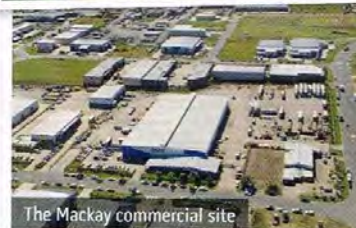
The Mackay commercial site
